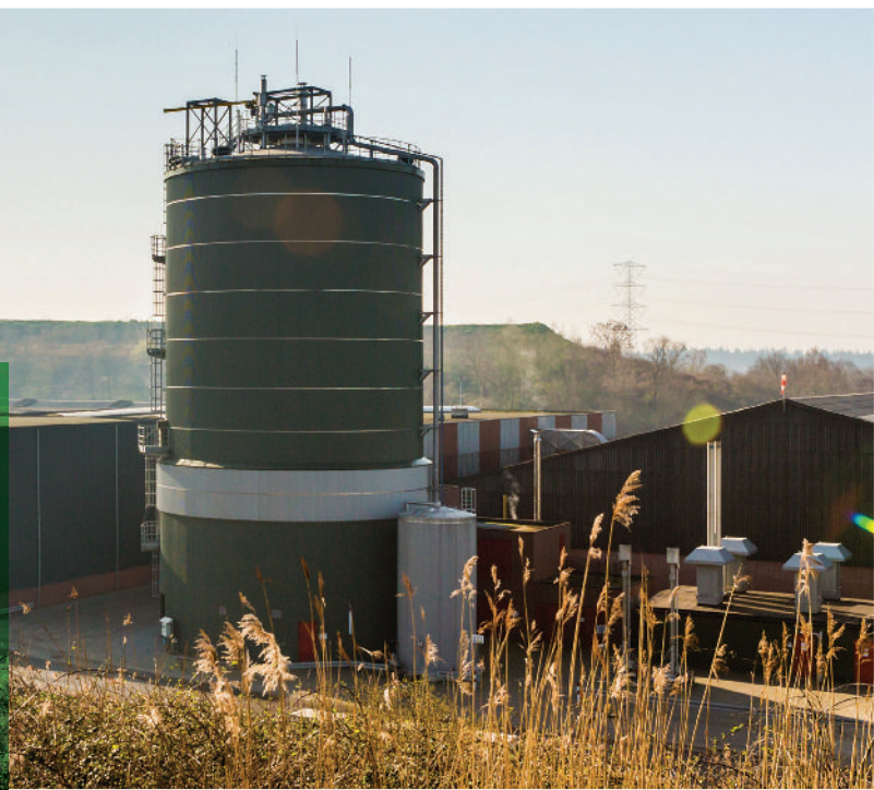
DRANCO partial stream digestion plant in Hengelo (The Netherlands)
